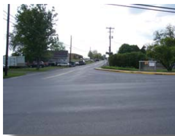
This intersection at North Corporation and Steelstown Road in Newville Borough illustrates an extremely wide turning radii and lack of sidewalks and curbs that makes crossing the street dangerous.
